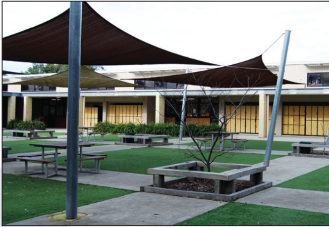
The new Year 10 classrooms
